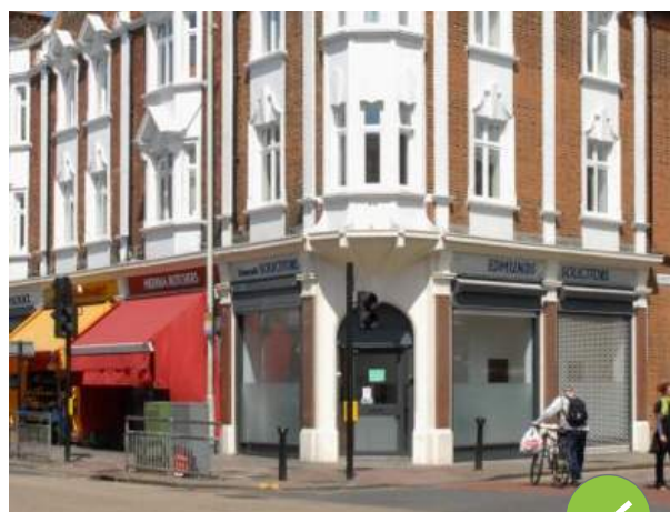
Double aspect frontage on a corner shop
