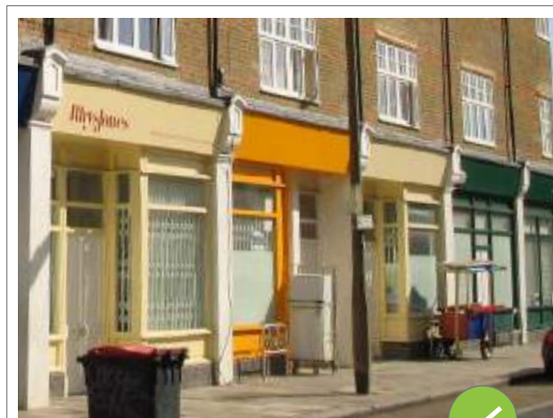
Internal shutters which don't obscure architectural features
