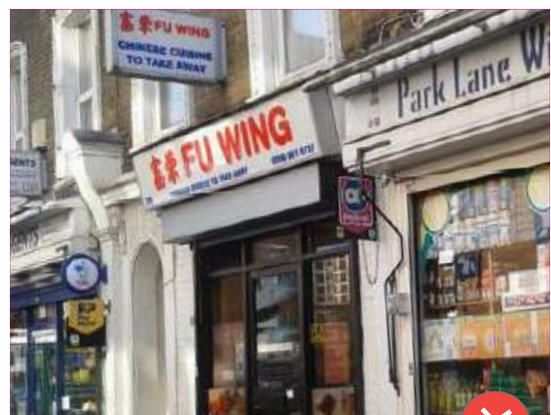
Illuminated box fascia's are not appropriate
